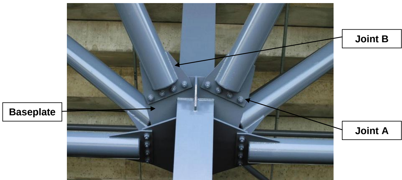
Figure 6: Steel Structure Connections
