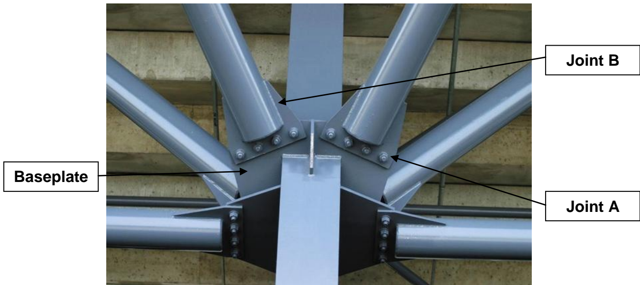
Figure 6: Steel Structure Connections
