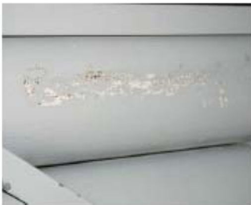
Figure 1: Corrosion
